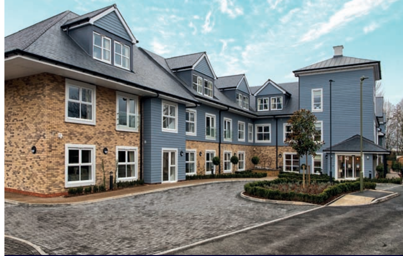
Located in Benson, near Wallingford
